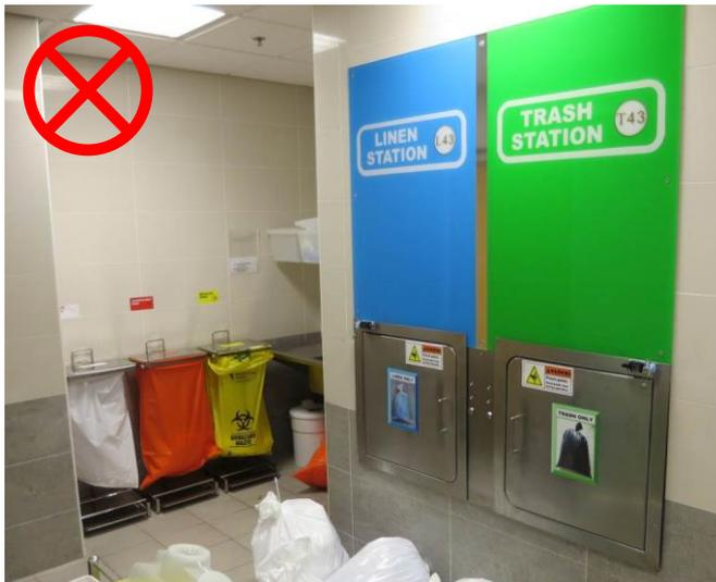
**Figure 16: Linen and Waste chutes are not permitted**
