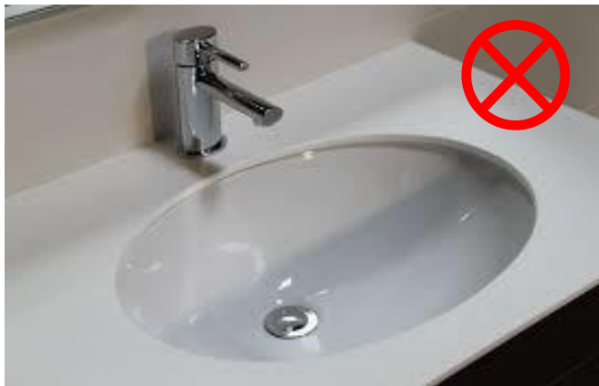
Figure 4: Under mount hand basin not recommended
