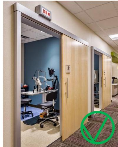
**Figure 26: Surface sliding doors permitted when meeting fire safety regulations**
